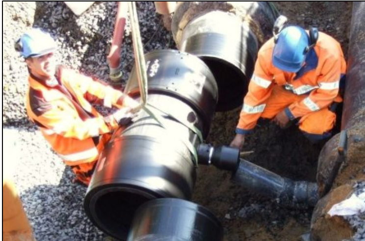
Figure 9B3: Maintenance work.
