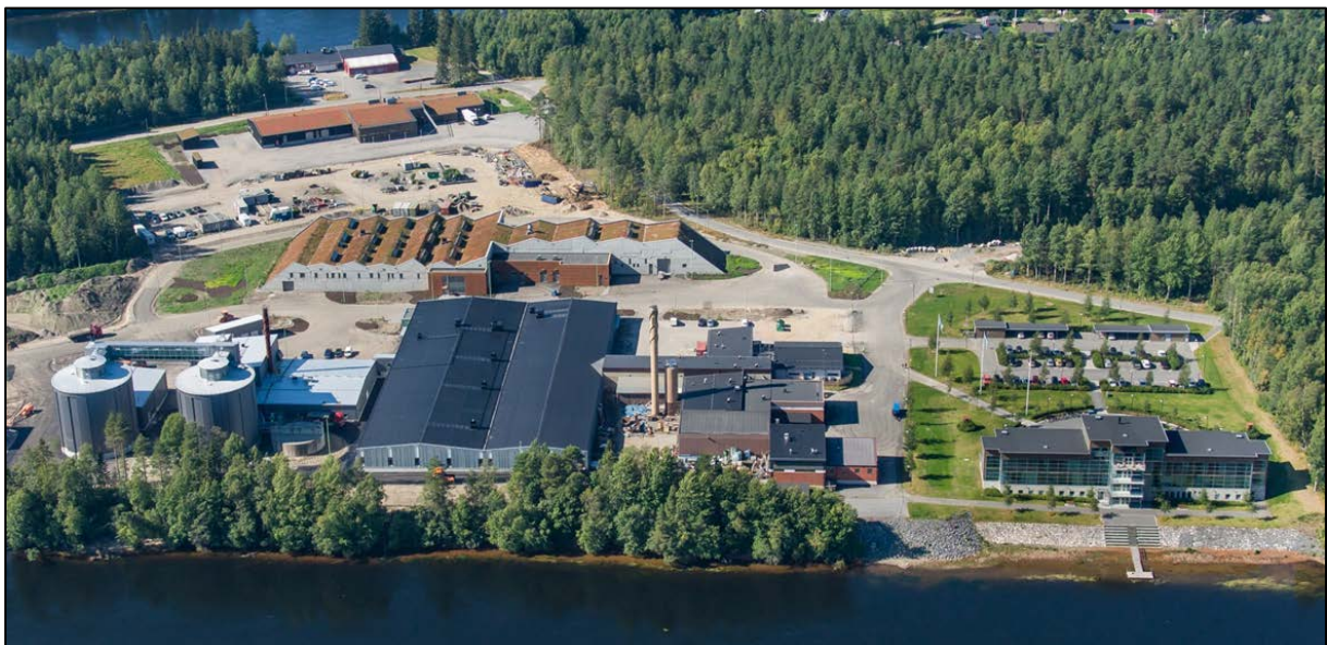
Figure 9B1: The new UWWTP at Ön in August 2015.
